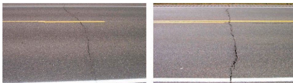
Figura 4-21: Fissuras transversais
